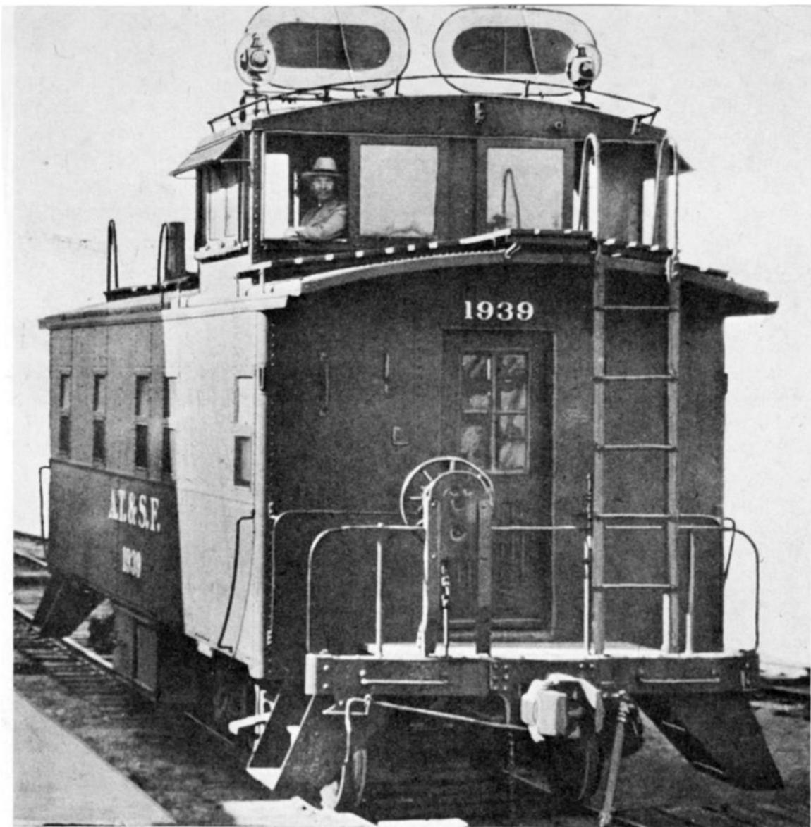
Ever see a way-car equipped with Marcum airbrake signal? Indicators would be in this position, crosswise to car, if a train were coupled ahead and brakes set.
